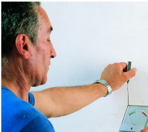
Checking gypsum plaster humidity
