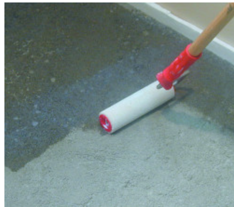
Applying Primer G with a roller
