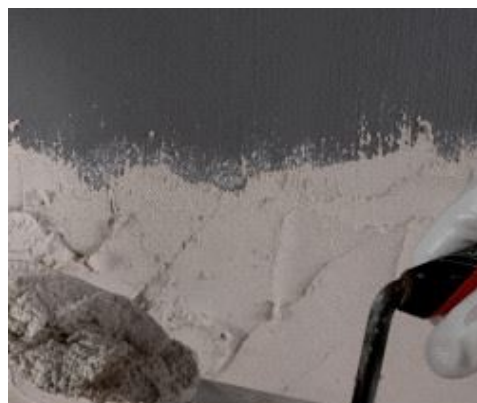
Application of render on Eco Prim Grip Plus
